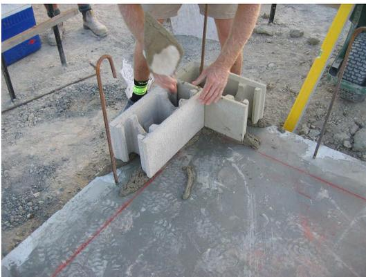
It will generally be necessary to set the first course of blocks in a mortar bed, but if the footing or base slab is precisely finished to an accurate level then this is not essential. Be aware however that if there is any unevenness or variation in level whatsoever it will be reflected throughout the entire height of the wall.
