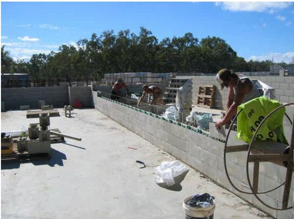
Use a string line stretched between the ends or corners of each length of wall to align the top corner of each block, and fill in each course of blocks maintaining tight perpend between all blocks. After the course is laid, install a connector at each perpend. Repeat this procedure on subsequent courses ensuring always that the perpend are tight and that the horizontal reinforcing bars are installed at the specified intervals.
