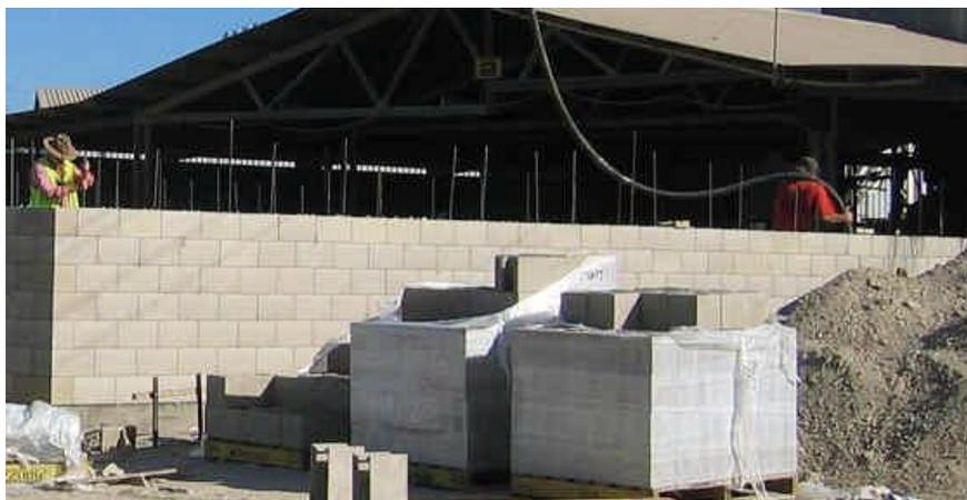
It is recommended that walls be grouted in maximum lifts of 1.4m (7 courses). As with any block wall, the higher the wall being grouted the greater the pressure of the wet grout and the greater the risk of a blow out during grouting.
