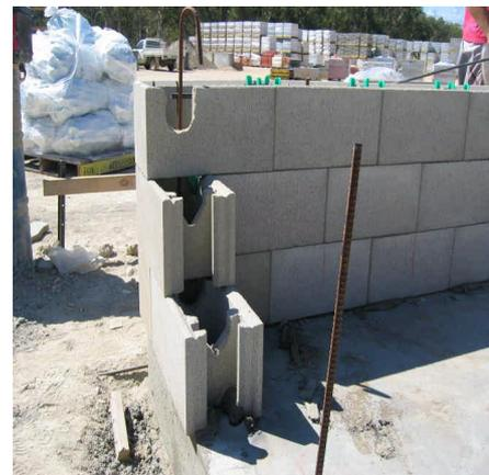
Build up the ends and corners of the walls true to a plumb line on all faces, ensuring all blocks are laid with tight perpend and ensuring all perpend are tied with plastic connectors. Install horizontal reinforcement as required by the engineer. Do not neglect to install corner bars and lap bars when building up ends and corners.
